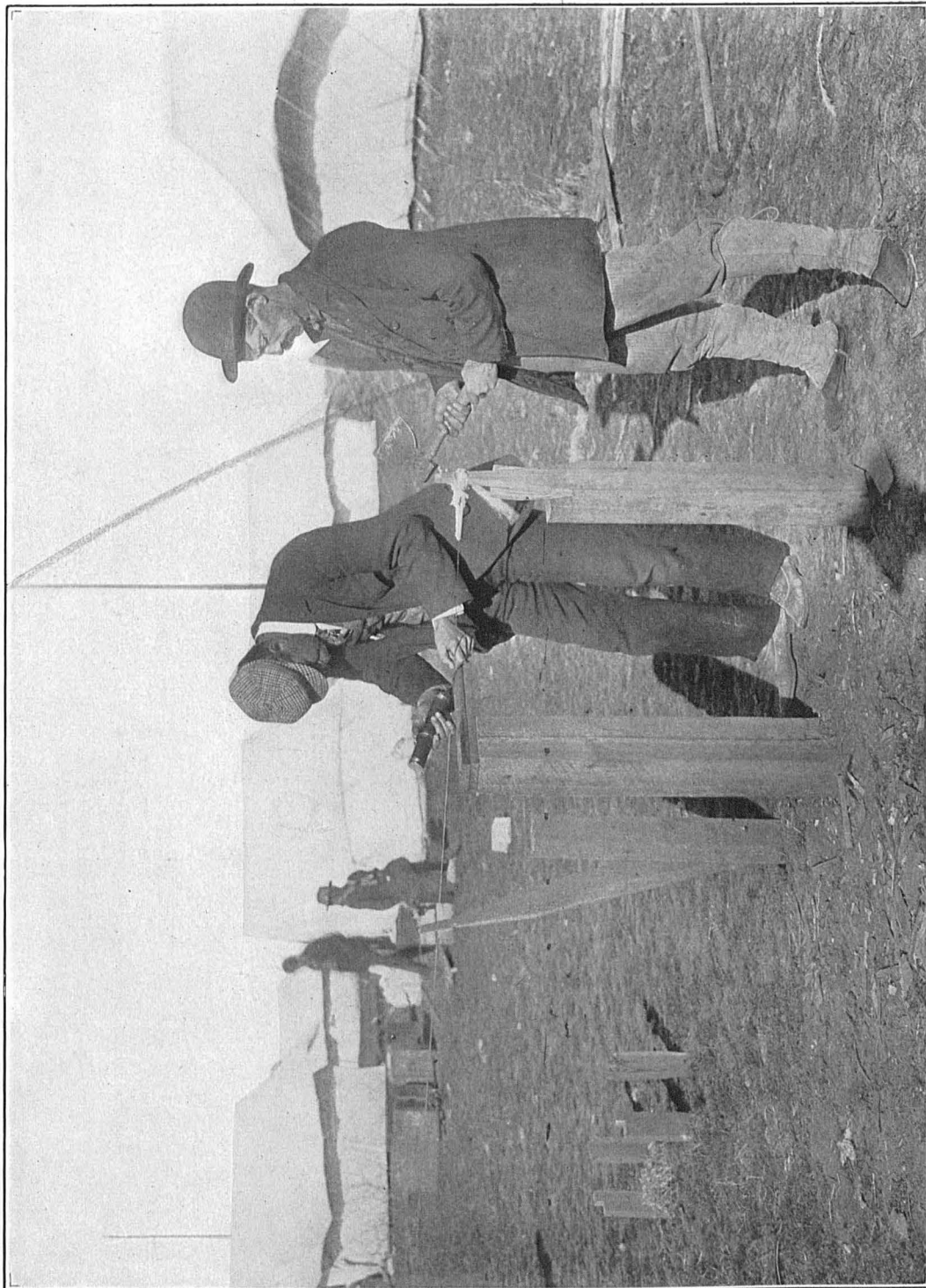
TAPE CONTACT AT MIDDLE OF COMPARATOR.
