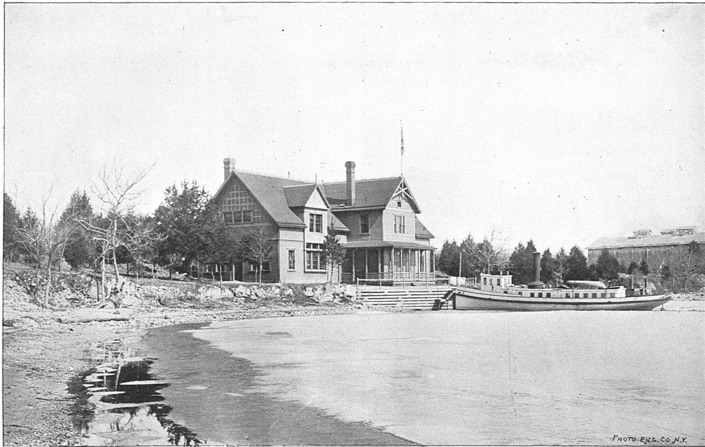
HATCHERY, WITH STEAMER SHEARWATER AT DOCK, PUT-IN BAY STATION, OHIO.
