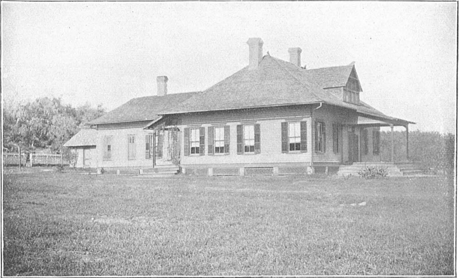
SAN MARCOS STATION, TEXAS—WEST SIDE OF SUPERINTENDENT S DWELLING.
