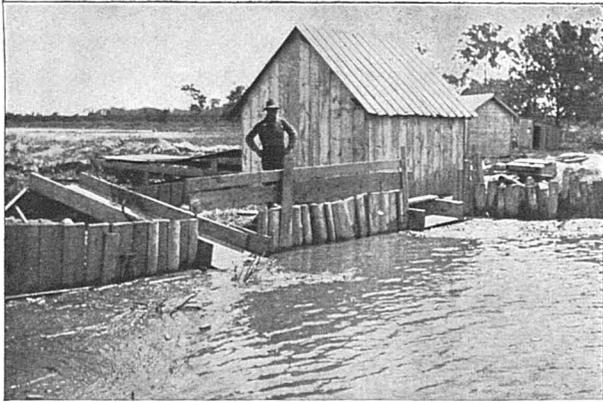
1. Dam and engine house of a carp pond at Port Clinton, Ohio. Carp are slid into the pond from the chute on the left; fresh water is received from the chute on the right, which comes through the engine house.
