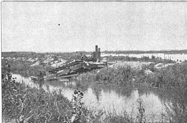
3. Supplementary engine and elevator for carrying water from dredge cut to pond, Monroe, Mich.
