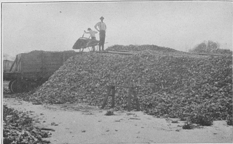
FIG. 2.—LOADING OYSTER SHELLS INTO CAR FOR USE IN BUILDING ROADS.
