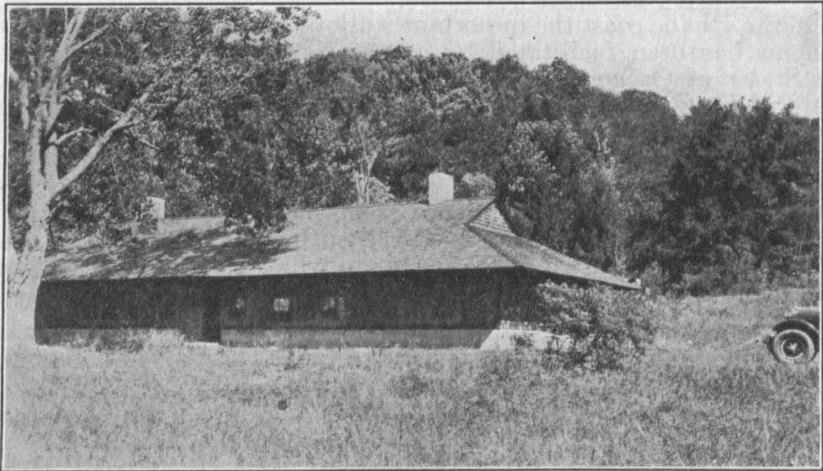
FIGURE 1.—Cooperative fish hatchery at Barneveld, N. Y.
