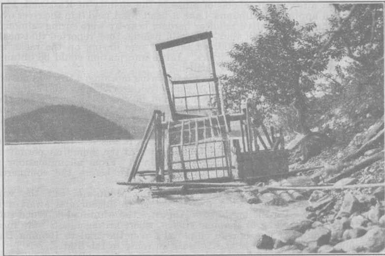
FIG. 2.—Native type of fish wheel on Copper River, Alaska
