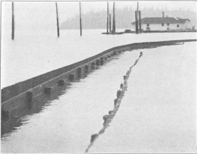
FIGURE 6.—Outside wooden wall protecting the diked area from crawfish
