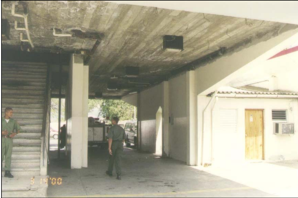
Fire Station Assessed for Disaster Resistance - Dominican Republic
