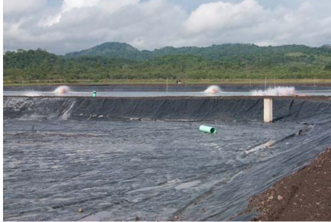
Lined Ponds With Aerators
