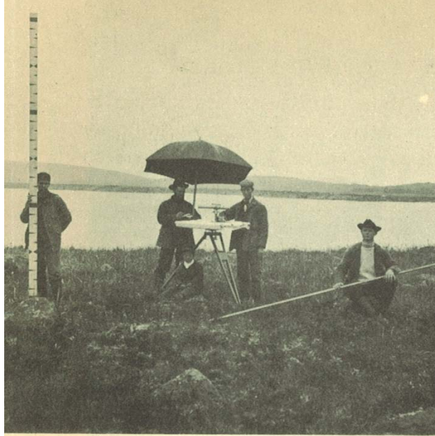
PHOTOGRAPH FROM COAST AND GEODETIC SURVEY, 1897. Topographic mapping party on St. Paul Island in Bering Sea. The author is at the plane table, with rod-men and recorder.
