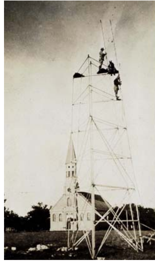
The oldest known photograph of a Bilby Tower being erected, 1928
