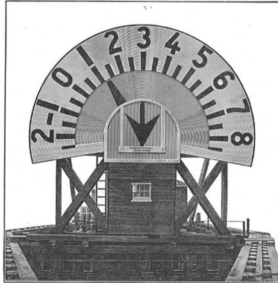
FIG. 5.—Tidal indicator, Delaware River, Delaware.
