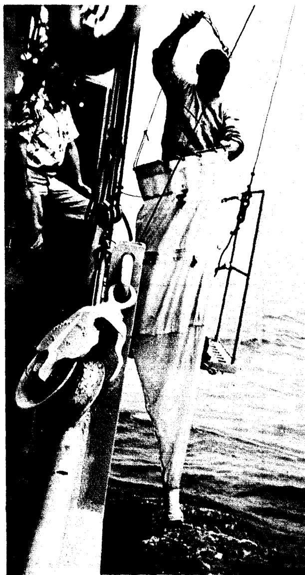
SETTING 1/2-METER TOW NET FROM RESEARCH VESSEL CISCO . THIS CLOSING NET IS USED TO STUDY THE VERTICAL DISTRIBUTION OF LARVAL FISH AND LARGER FOOD ORGANISMS
