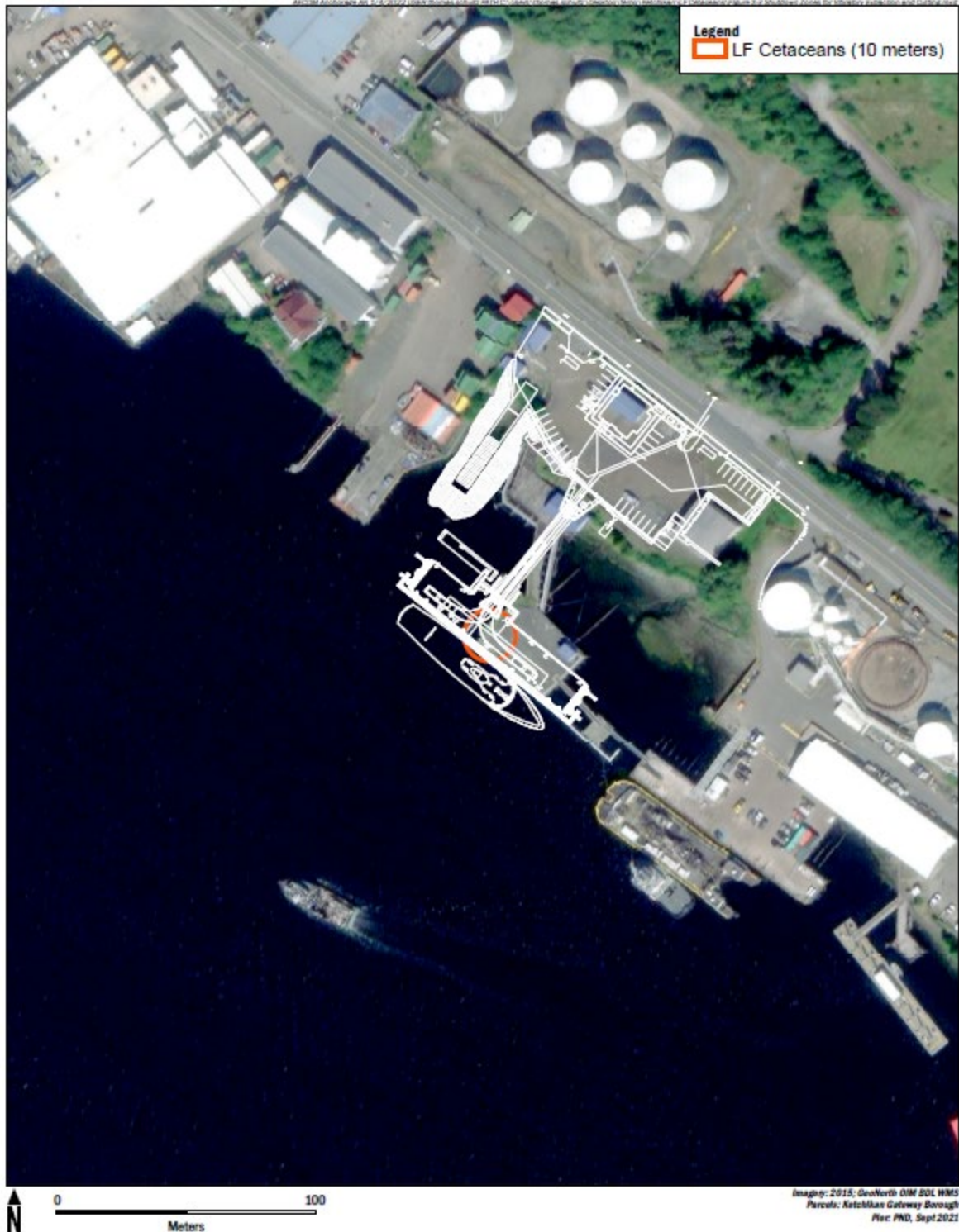
Figure 5. Example of a 10-m shutdown zone for pile removal (direct pull, vibratory extraction, pile clipping) and other in-water construction activities (figure prepared by AECOM). Shutdown zones will be centered on the pile being installed and may differ from what is depicted in this figure, depending on the location of the pile.
