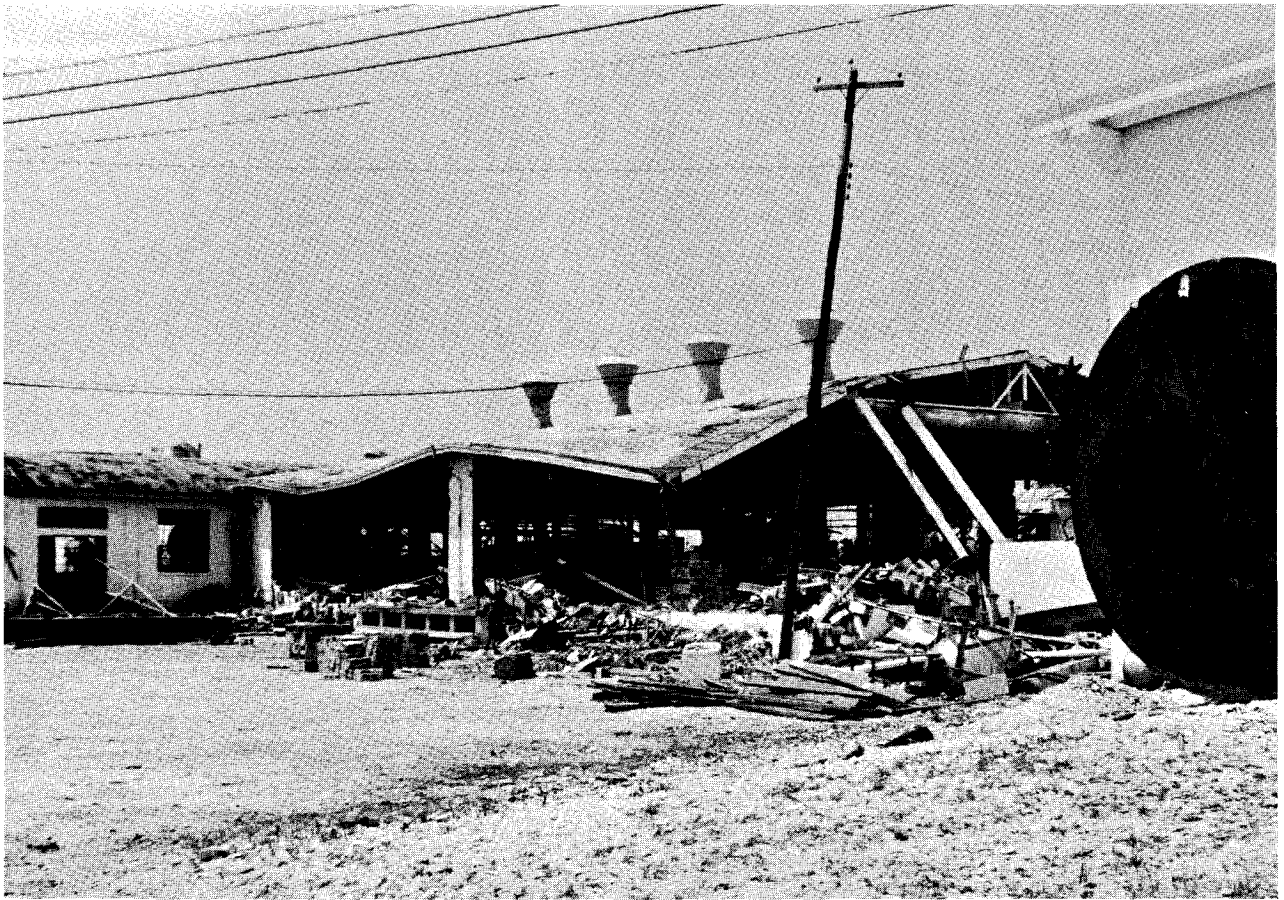
Figure 1. Destruction to the Biloxi seafood processing industry caused by Hurricane Camille.
