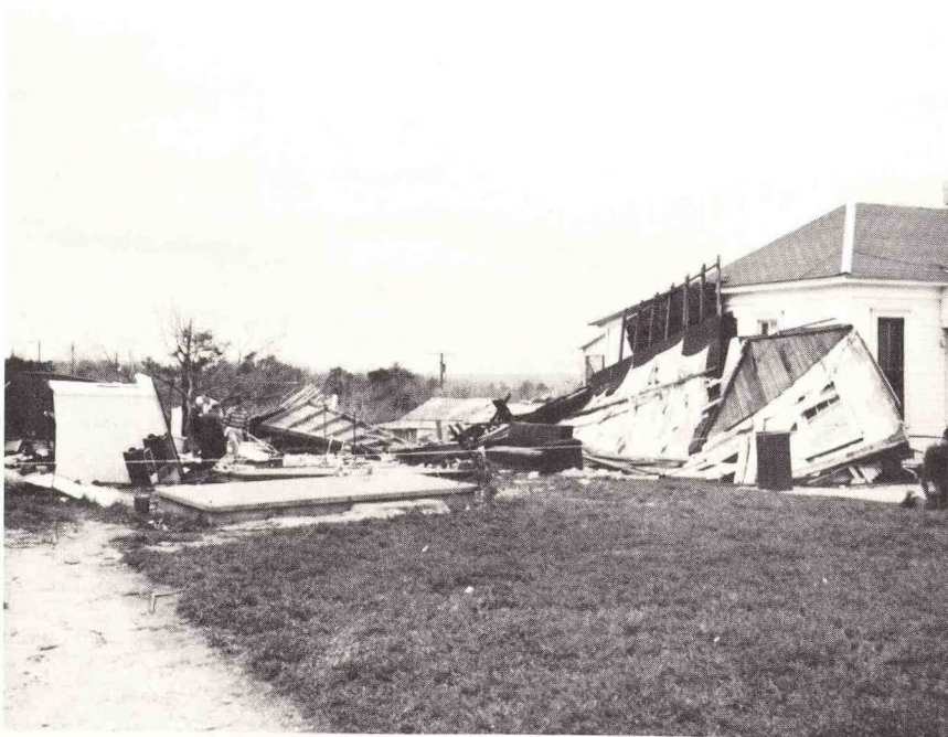
FIGURE 4.—Complete destruction of wooden house constructed with no studs in the outside walls. Undamaged house next door was of approximately the same age.
