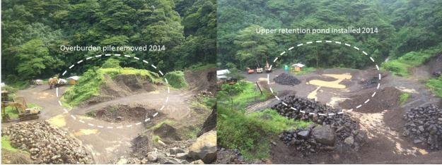
Figure 6. Pictures of the Upper Operational Area/Excavation Platform before (left) and after the installation of the Upper Retention Pond. A similar retention pond is also installed at the Lower Operational Area (not shown).
