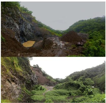
Figure 5. Pictures of the Excavation Platform before (2012, top) and after (2014, bottom) vegetation overgrowth of overburden piles. The groundwater seep is evident in the muddy puddle in the top picture. The groundwater diversion routed this flow to the right in the picture, into the stream before it could erode the Platform surfaces. Pictures taken by Alex Messina.
