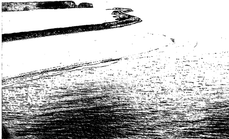
Figure 124. Glass Breakwater. Orote Island and Peninsula are in the background. The Luminao Reef forms a broad platform on the seaward side of the breakwater.
