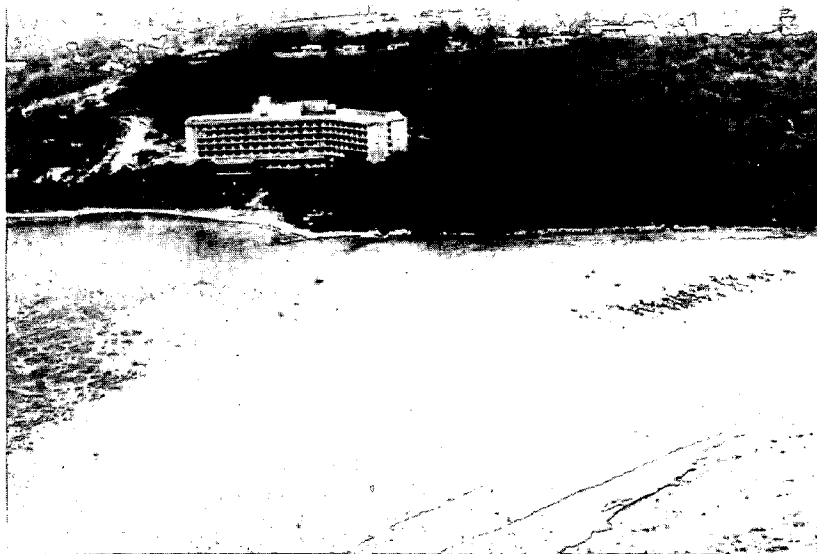
Figure 98. Hilton Hotel and steep limestone slopes and cliffs border the south end of Tumon Bay.
