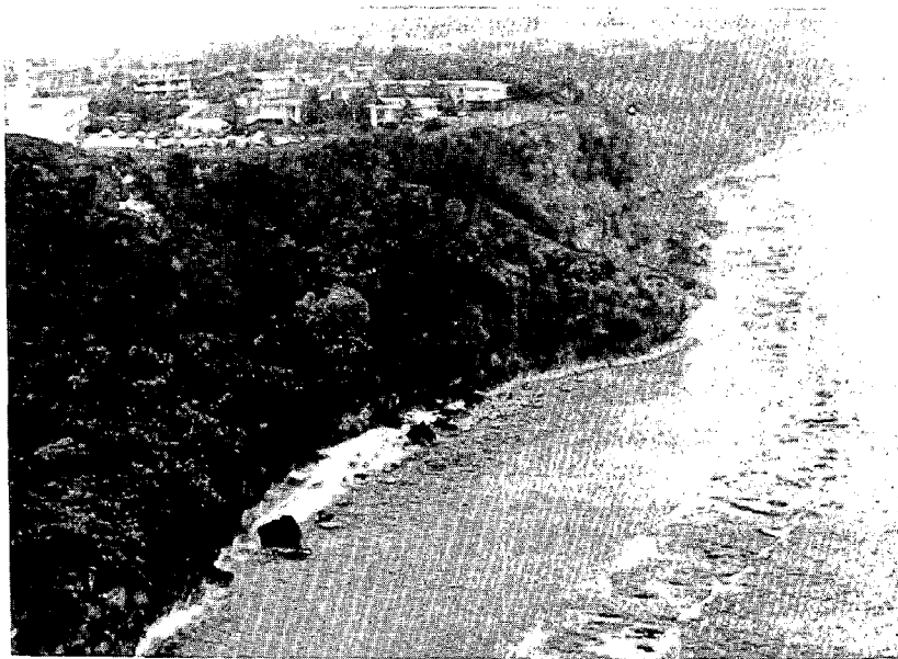
Figure 102. The narrow reef flat at Ypao Point grades into a narrow cut bench. On the plateau above is the Guam Memorial Hospital. Note large limestone block from which reef-flat transect was made.
