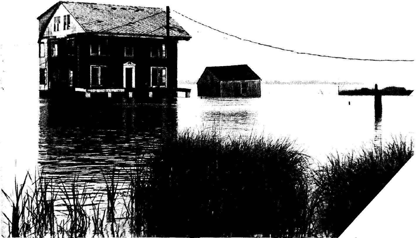
Subsidence. Baytown, Texas.
