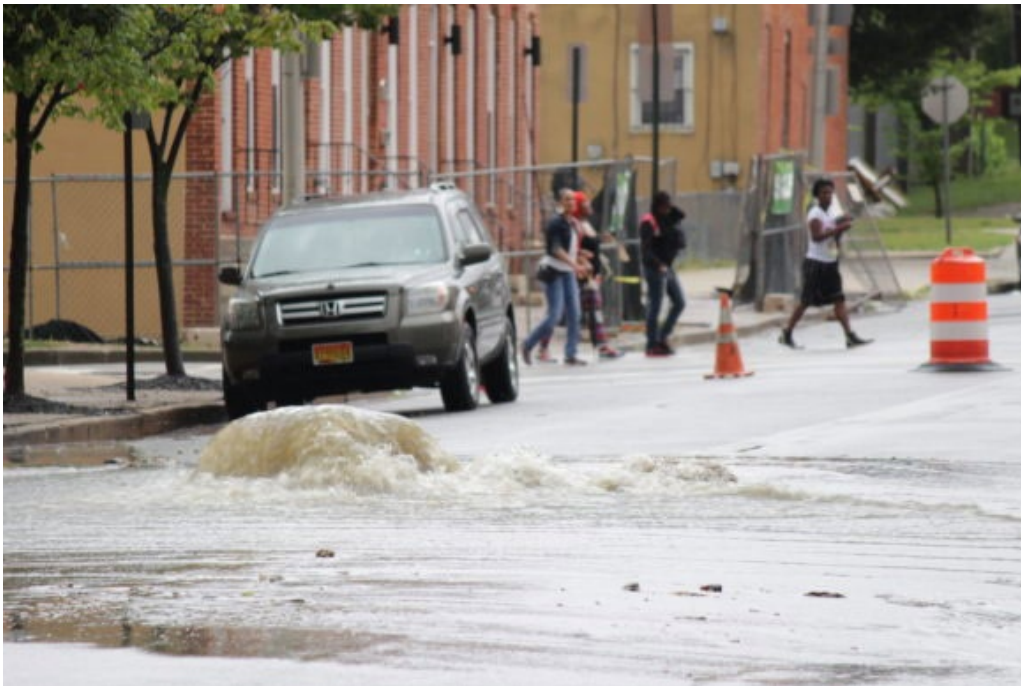
Figure 48. Backflow from a manhole in Baltimore. Credit: Blue Water Baltimore.
