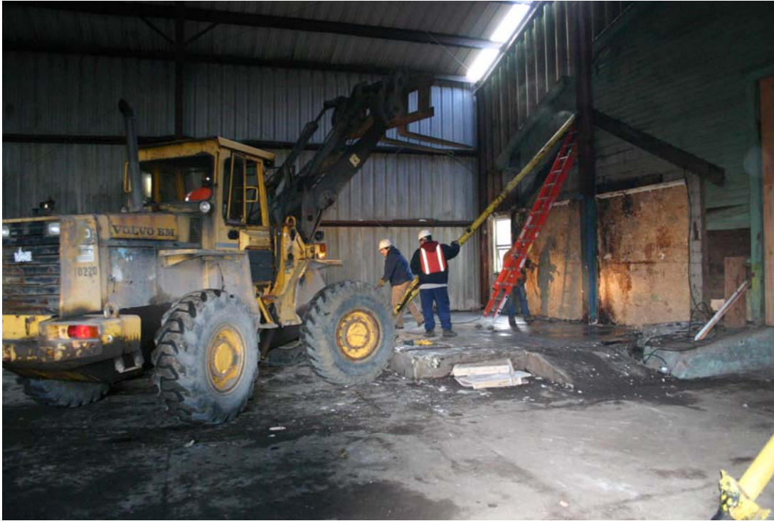
Figure 8. Bracing a frame of the Connector Building, October 2004
