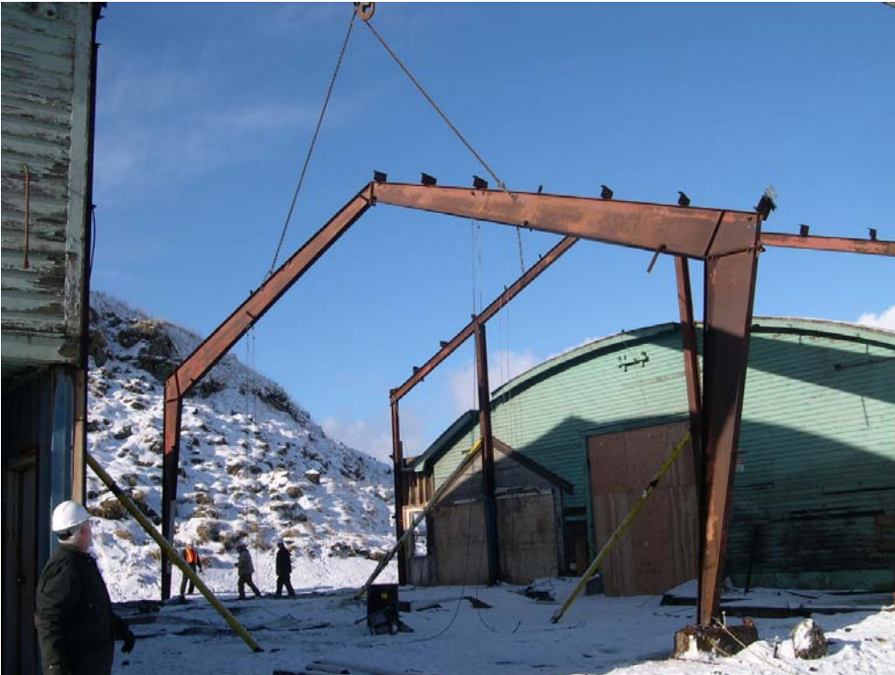
Figure 15. Removal of the center frame
