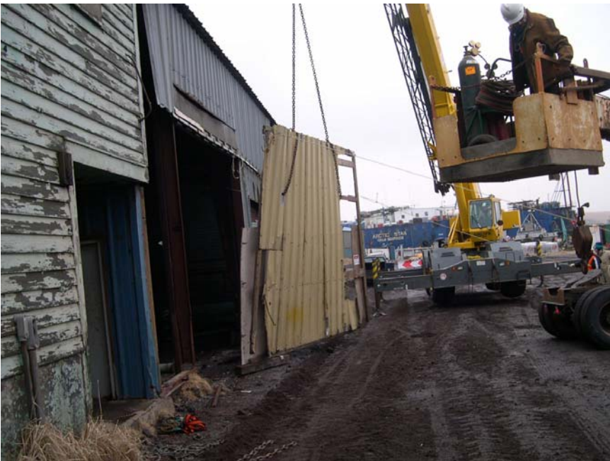
Figure 11. Removal of the sliding door, February 2005
