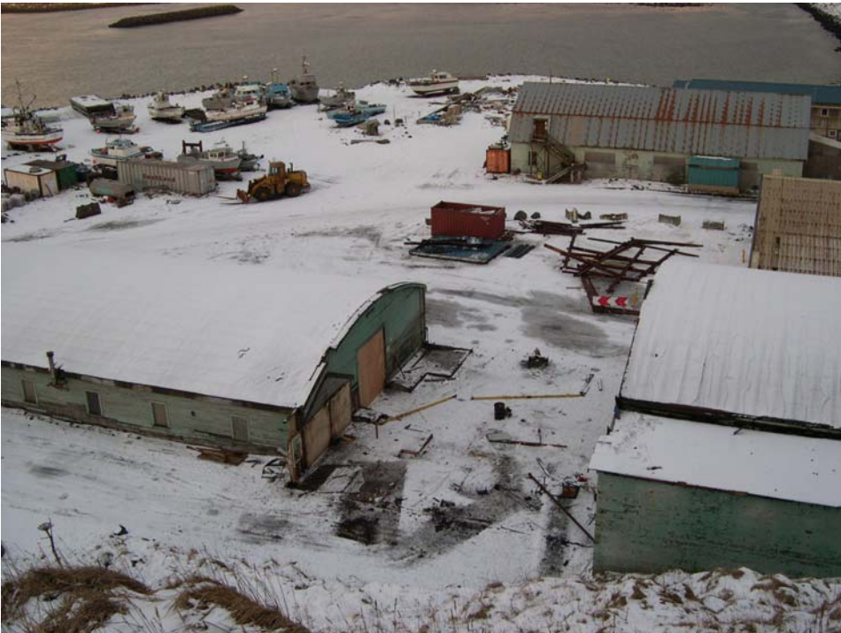
Figure 17. Aerial view of the area after the Connector Building demolition
