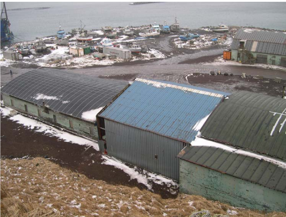
Figure 5. Aerial view of the Connector Building before demolition, February 2005
