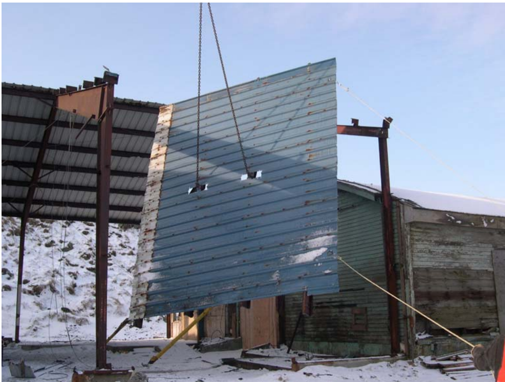
Figure 13. Removal of a roof section with the Grove crane
