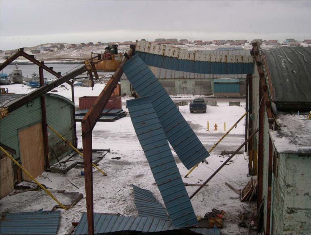
Figure 14. Removal of roof sections without the crane
