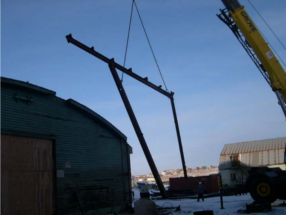
Figure 16. Removal of a section of a side frame
