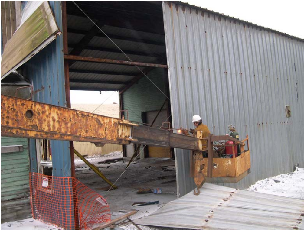
Figure 12. Removal of the west wall
