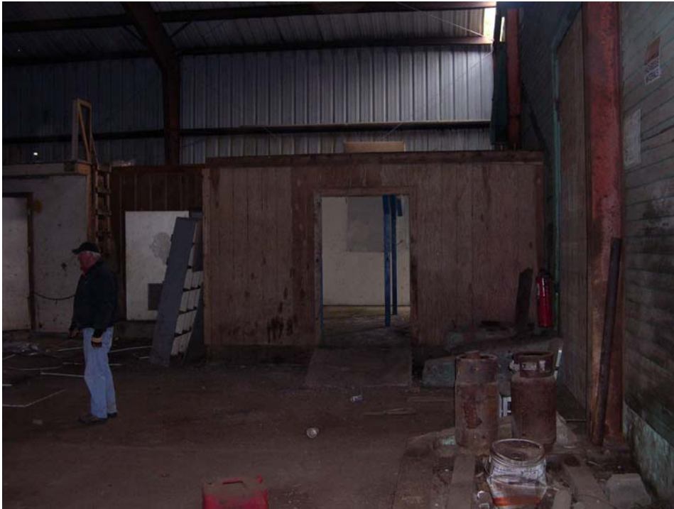
Figure 6. The wooden structure inside the Connector Building
