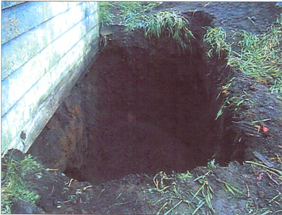
Figure 6. Extents of excavation
