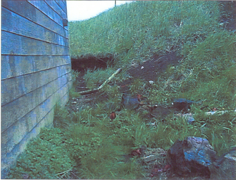
Figure 5. OMT excavation area prior to excavation activities
