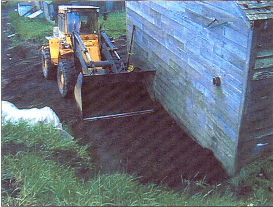
Figure 7. Final grading of clean backfill
