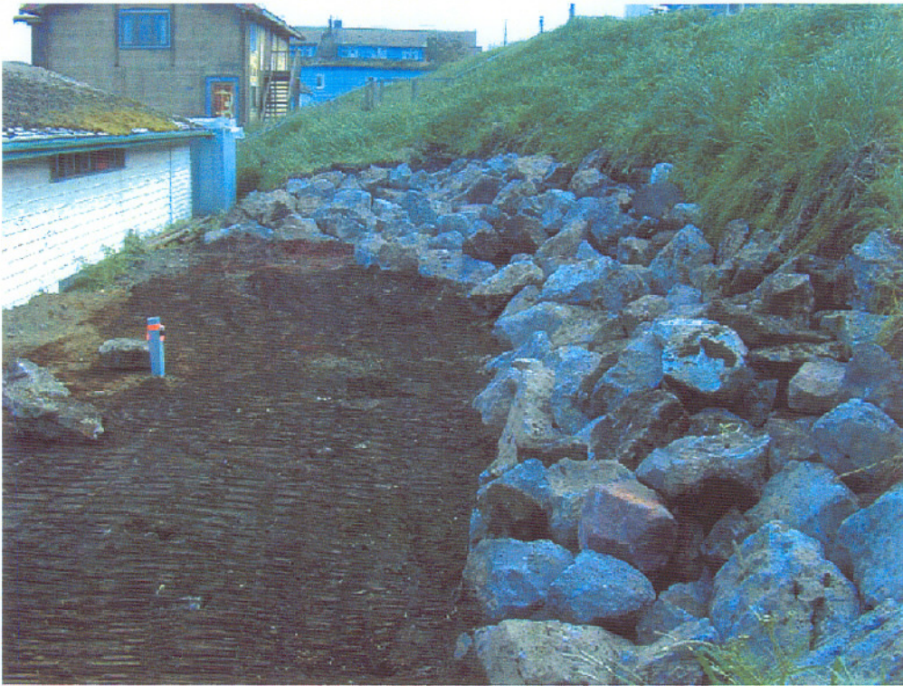
Figure 9. Final grade and rock wall to prevent erosion.
