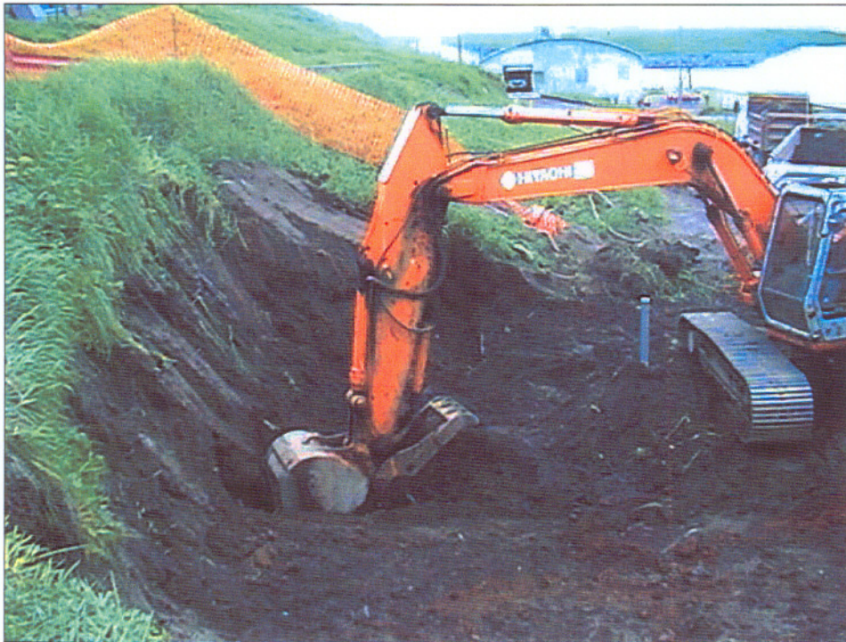
Figure 6. Excavating petroleum contaminated soils northwest of Duna's Kitchen
