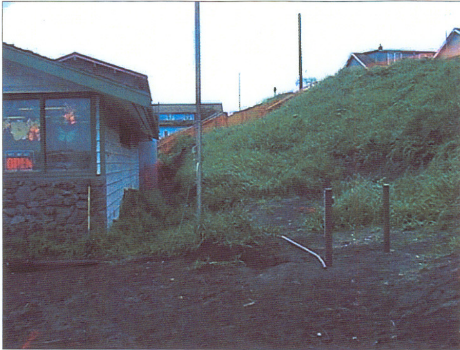
Figure 5. Former Power Plant site prior to excavation
