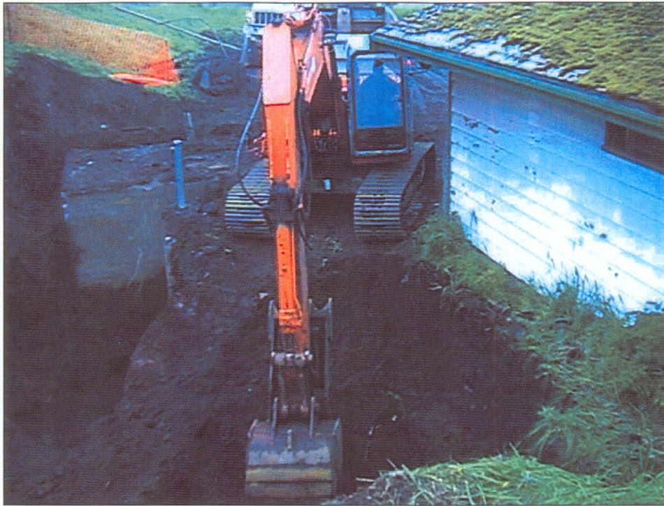
Figure 7. Excavation of petroleum contaminated soils west and south of Duna's Kitchen
