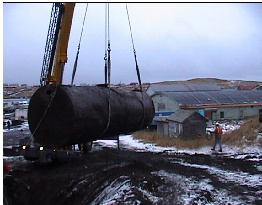
Figure 9. Underground storage tank removal
