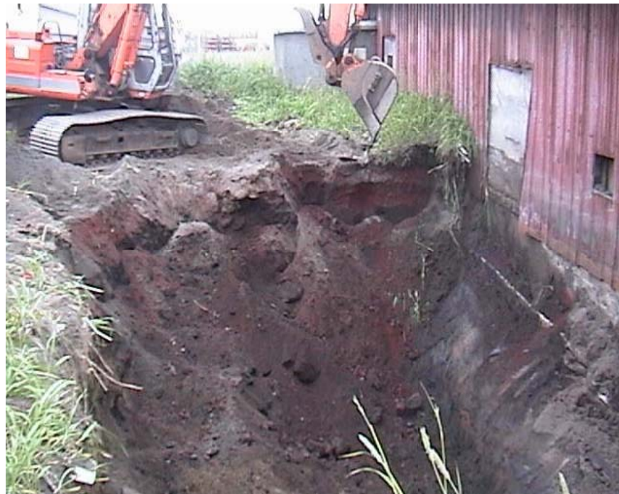
Figure 5. Excavation of Area 1, Phase I
