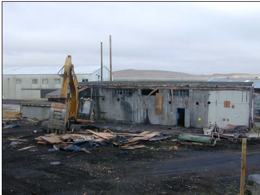
Figure 7. Demolition of the south side of the Decommissioned Power Plant
