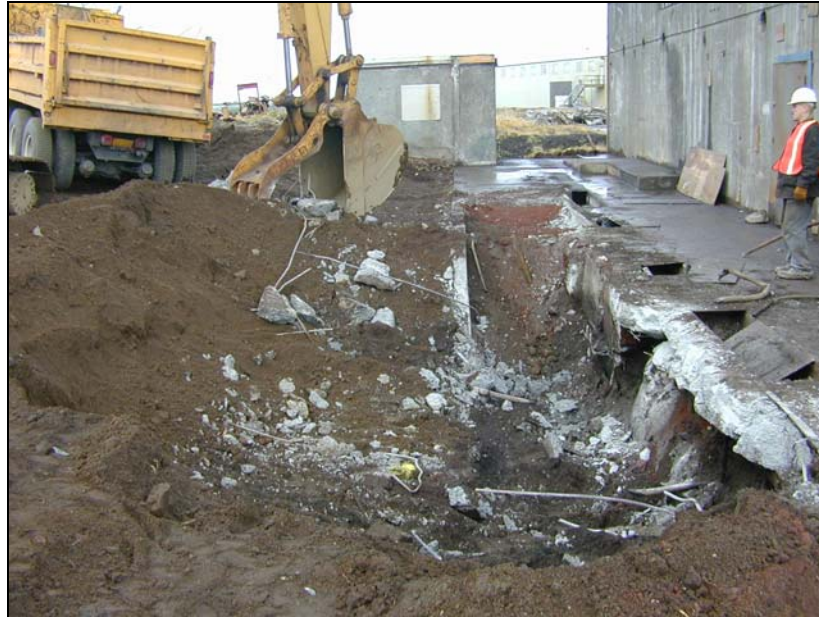
Figure 8. Removal of the Decommissioned Power Plant's concrete foundation
