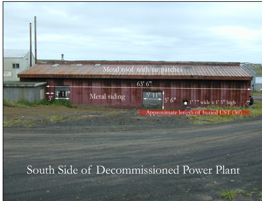
Figure 4. Decommissioned Power Plant
