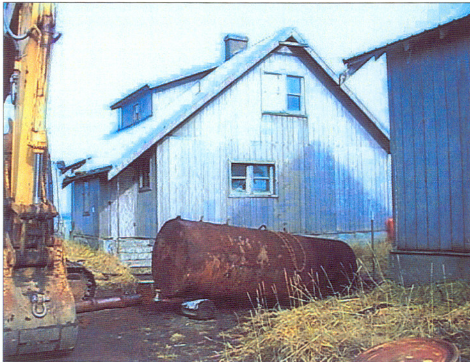
Figure 7. Removed 1000-gallon UST
