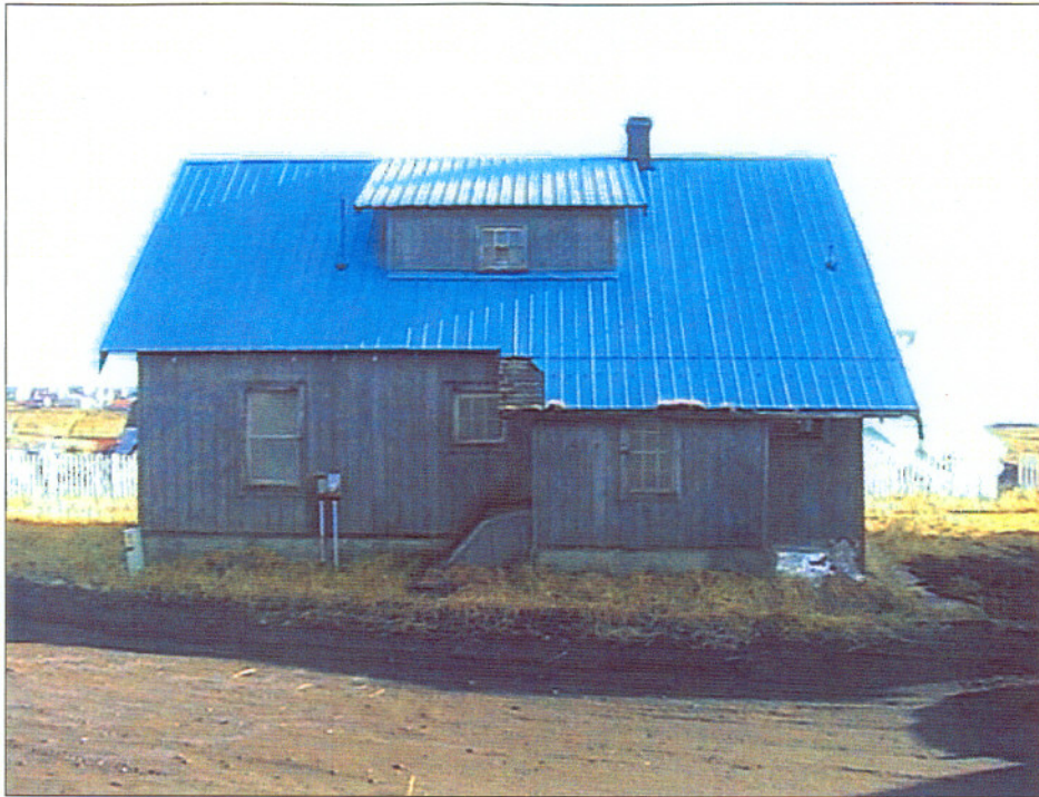
Figure 4. House 101, general view
