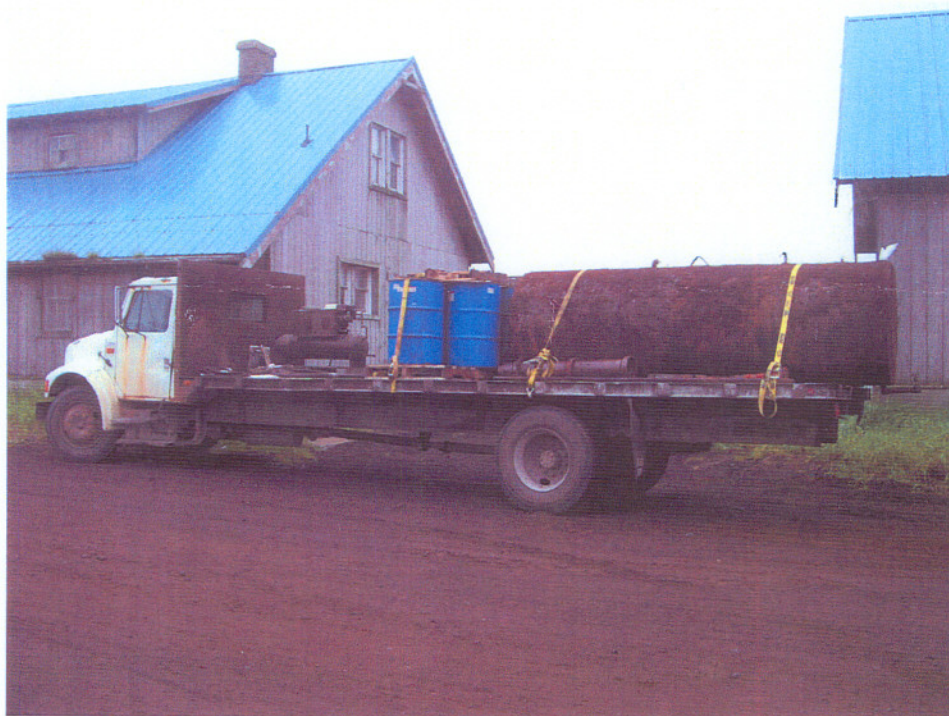
Figure 5. The underground storage tank removed from House 102.
