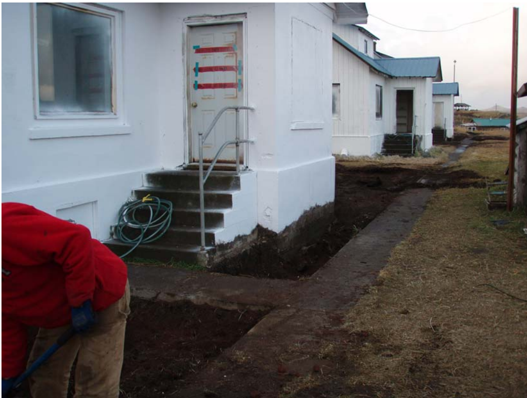
Photo 12. NTPA Site 60. Richard Warner and Excavation, East Side, TH103. NOAA. 10/2006.
