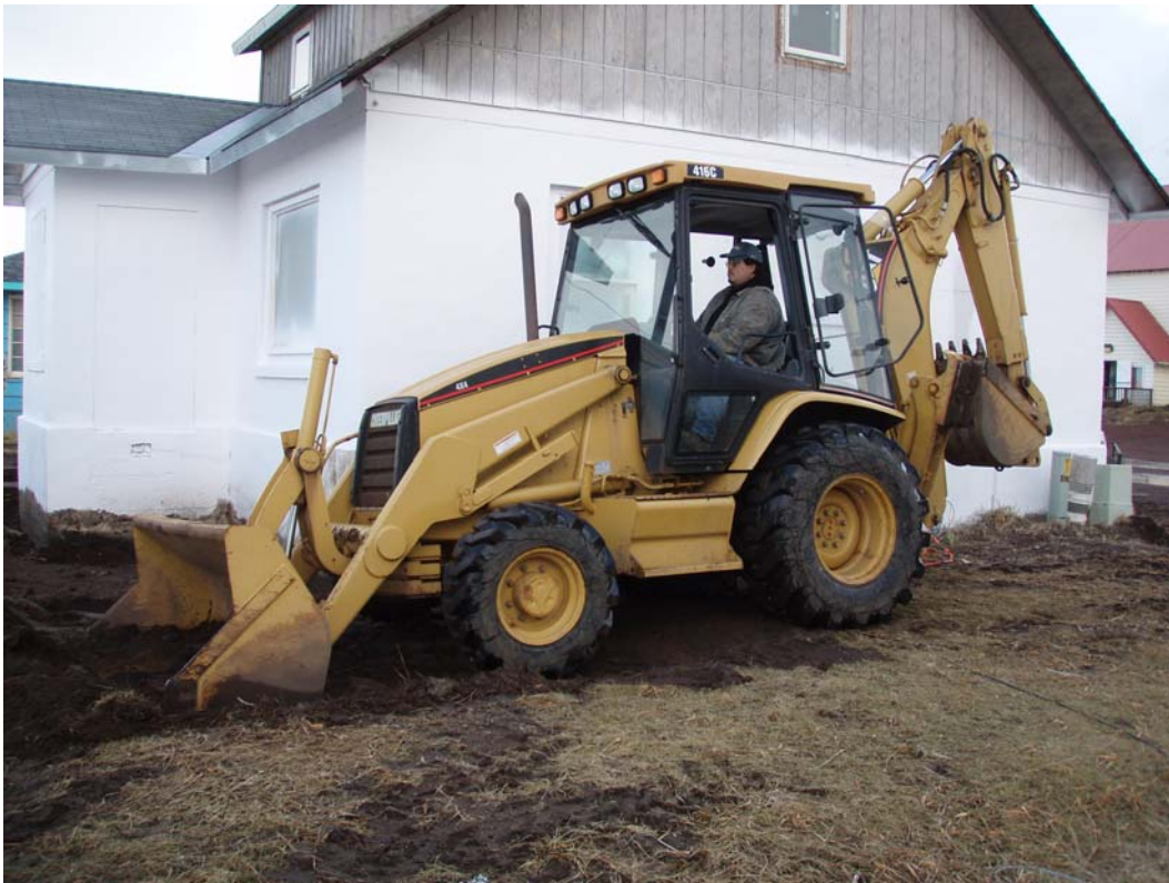
Photo 14. NTPA Site 60. Nick Kozloff Loading Temporary Stockpile, NE Corner, TH103. NOAA. 10/2006.
