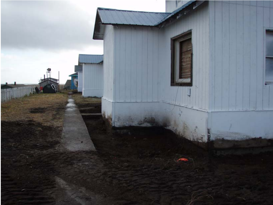
Photo 11. NTPA Site 60. Excavation, NE and East Sides, TH101. NOAA. 10/2006.
