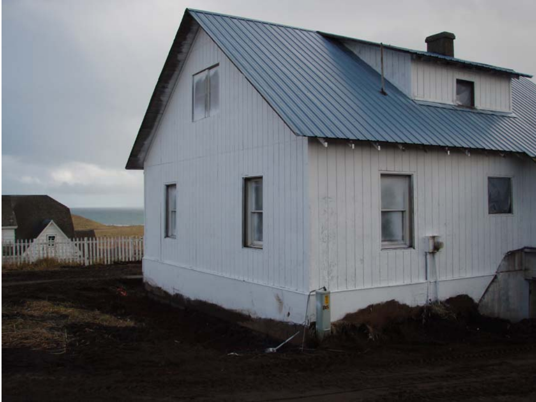
Photo 9. NTPA Site 60. Excavation and Buried Telephone Lines, NW Corner,TH101. NOAA. 10/2006.
