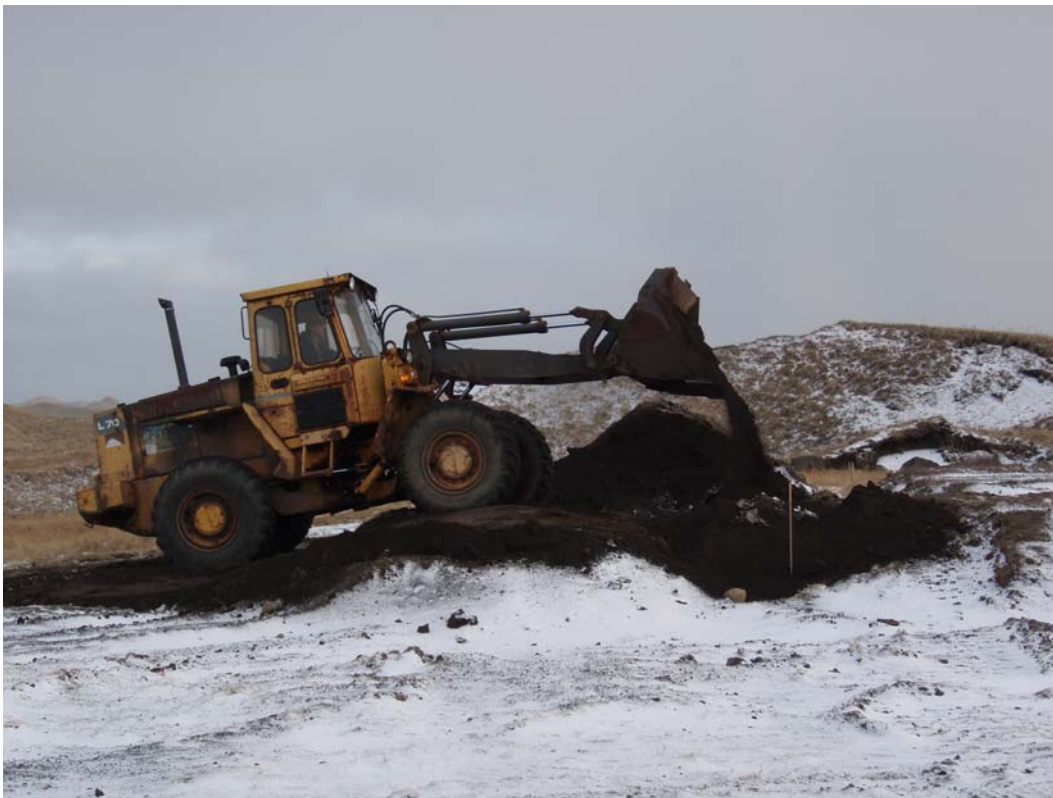
Photo 18. NTPA Site 60. Frank Shane Capping Disposal Pits, Landfill Cell C, Tract 42. NOAA. 12/2006.
