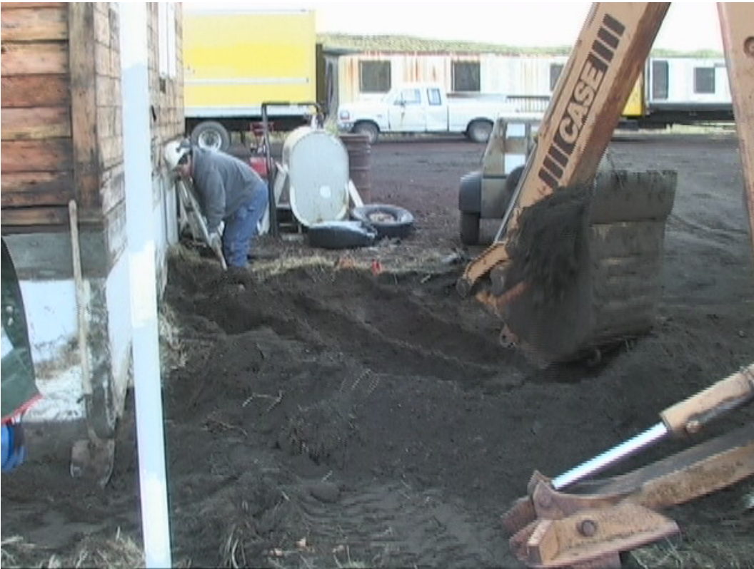
Photo 8. NTPA Site 60. Ray Beeter and Nick Kozloff Excavating Soil, Duplex. NOAA. 10/2006.
