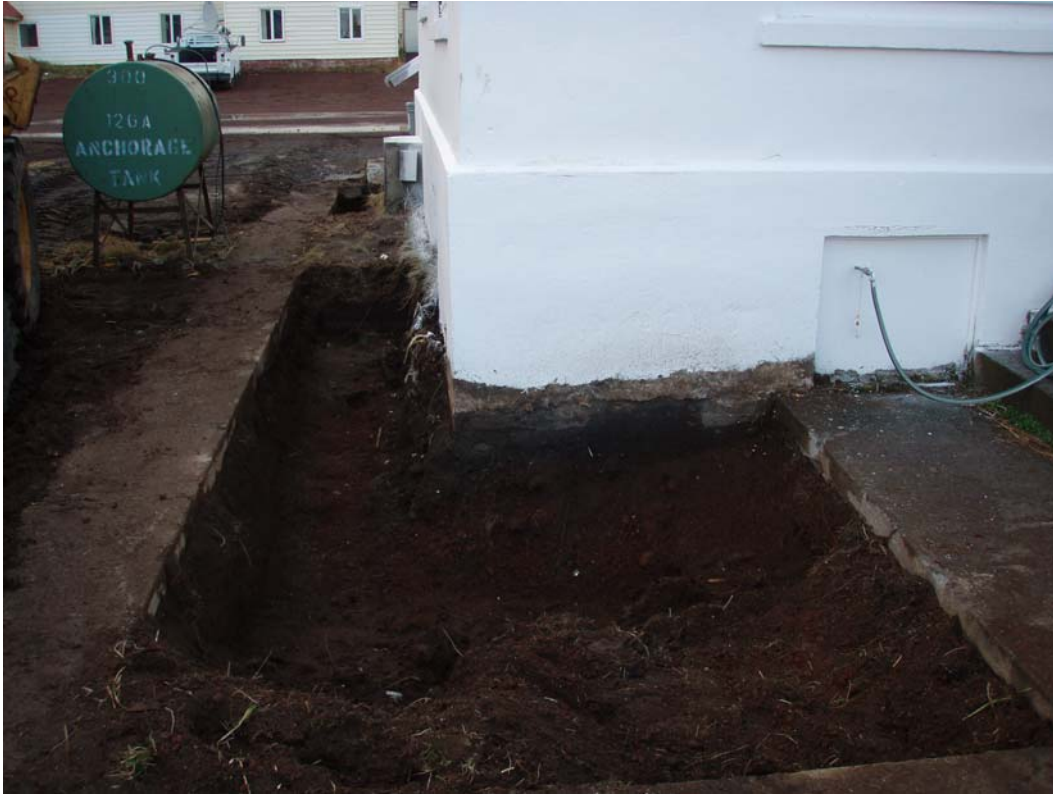
Photo 13. NTPA Site 60. Excavation Near AST, South Side, TH103. NOAA. 10/2006.
