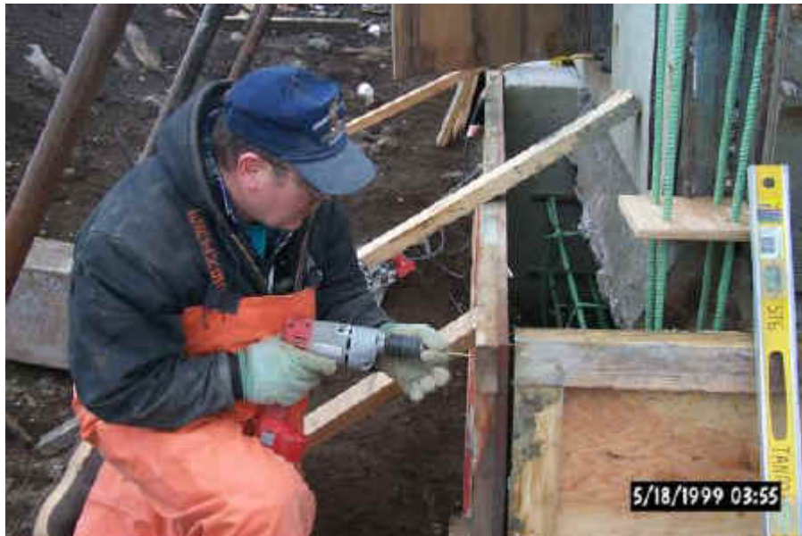
Putting forms together for grade beam.
