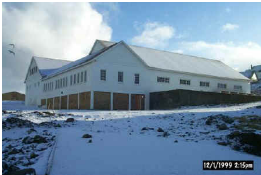
Finished Project. Frost on the roof is covering the cedar shingles which are the same as the ones on the exterior of the blubber house basement infill panels.
