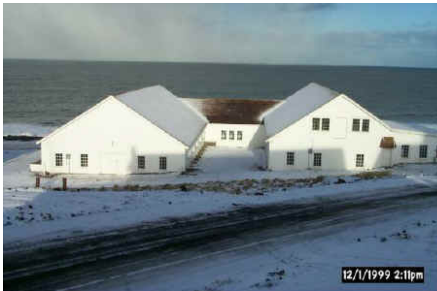
View of seal plant from the south.
