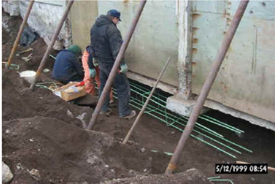
Figure 3. Construction of the Perimeter Grade Beam
