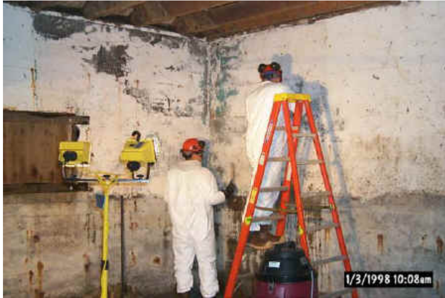
Figure 7. Lead Paint Removal
