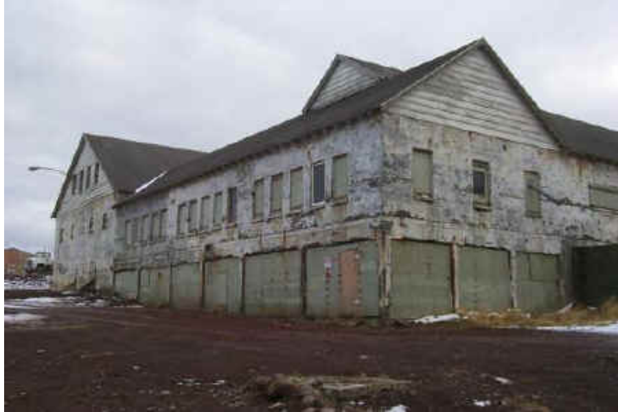
Picture of the Seal Plant before any work began in 1998.
