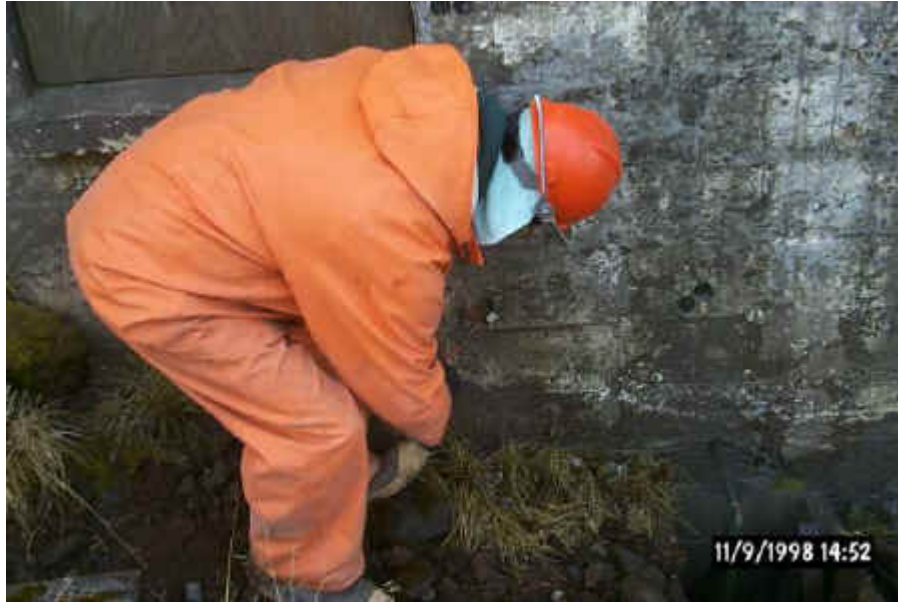
Figure 10. Wire Tie Removal
