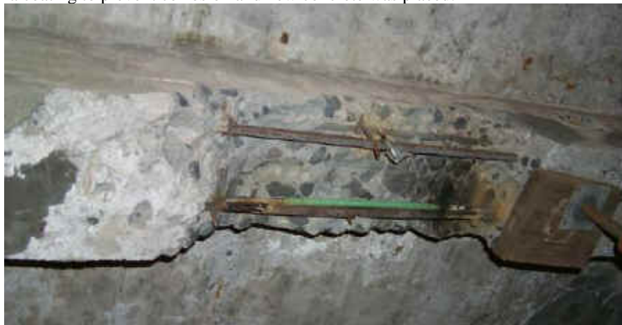
Figure 4. New Rebar for the Blubber House Slab and Support Beams
