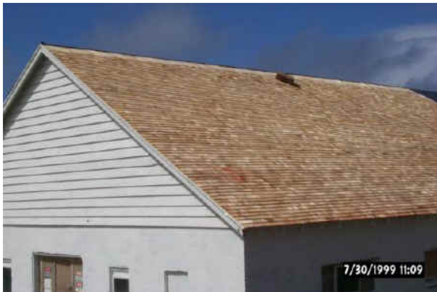
Close up of new cedar shingles.
