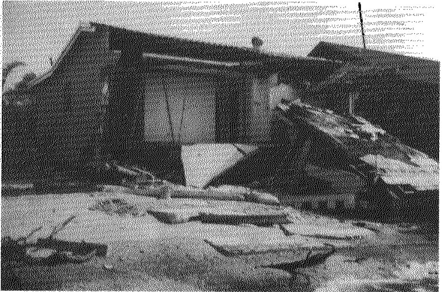
Figure 9-A. Hurricane Juan (1985) damage. (From Clark, 1986a.)
