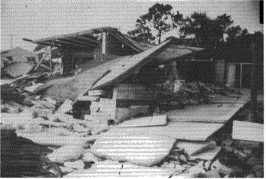
Figure 10-A. Hurricane Kate (1985) damage. (From Clark, 1986b.)
