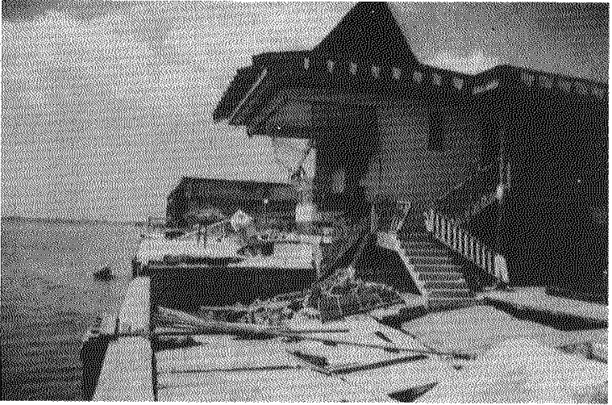
Figure 8. Hurricane Elena (1985) damage. (From Clark, 1986a.)
