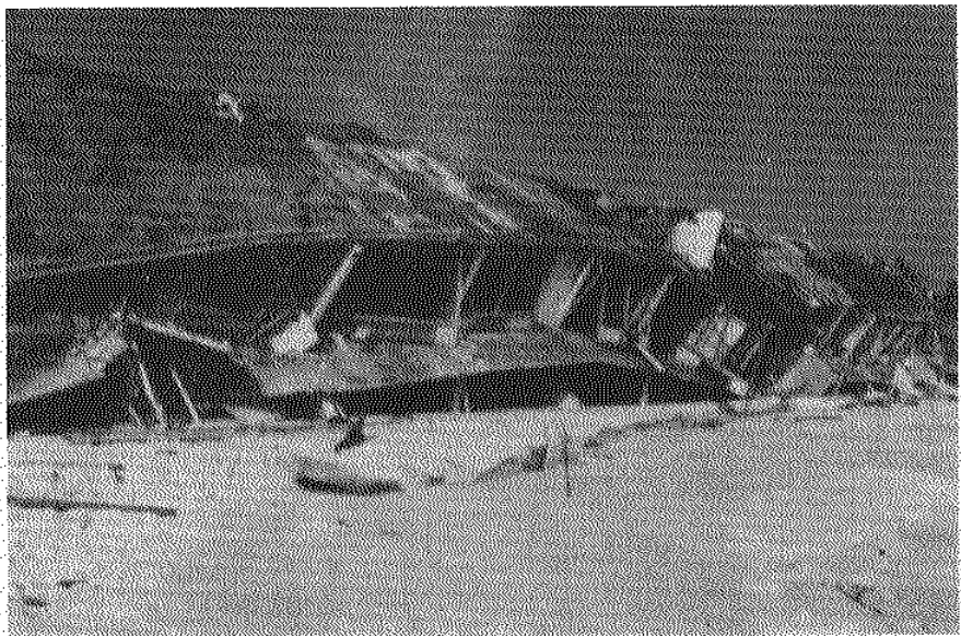
Figure 9-C. Hurricane Juan (1985) damage. (From Clark, 1986a.)
