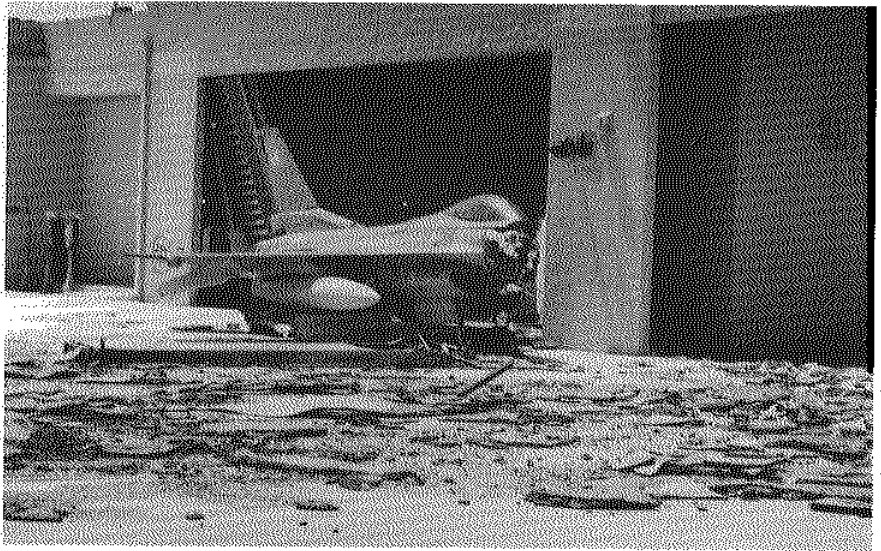
Figure 11-J. Homestead AFB, Hurricane Andrew. (Courtesy of Larry Floyd.)
