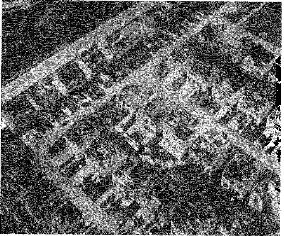
Figure 11-F. The roof and the hurricane. (U.S. Army Corps of Engineers, 1993.)
