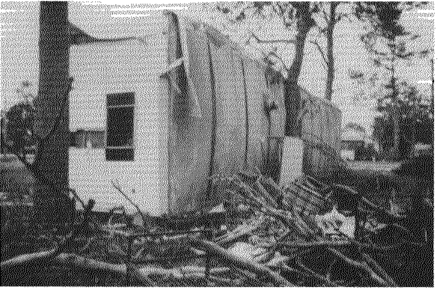
Figure 10-B. Hurricane Kate (1985) damage. (From Clark, 1986b.)
