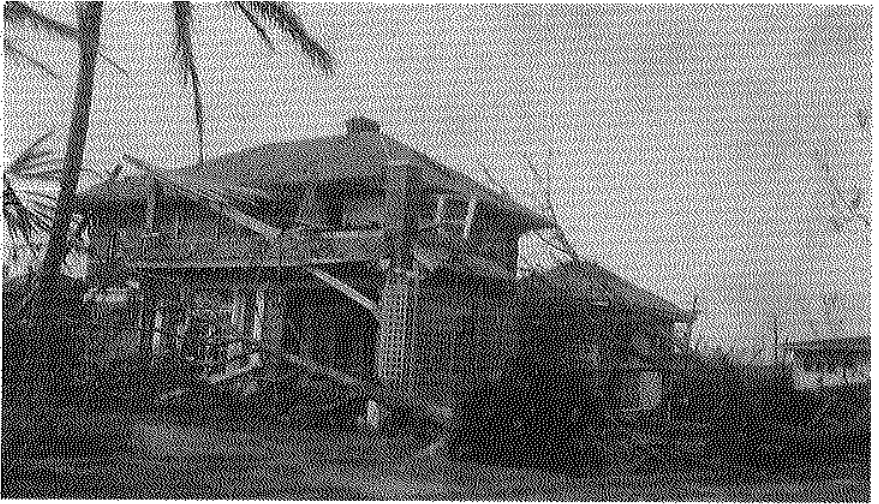
Figure 1-G. A damaged home, 1926 Miami Hurricane. (Courtesy of Richard Clark.)
