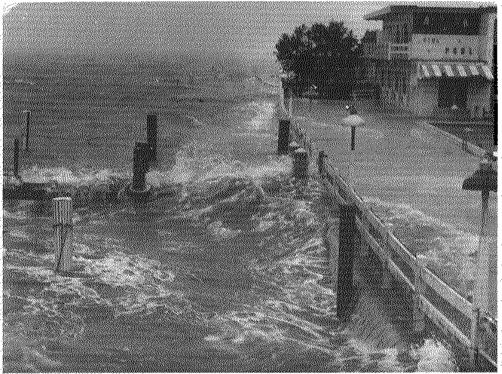
Figure 4-A. Hurricane Donna. Even though Hurricane Donna did not strike Miami, this photograph shows typical damage along the Dade County shoreline. (Courtesy of National Hurricane Center.)
