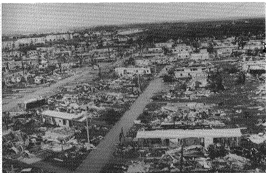
Figure 11-G. Mobil home damage, Hurricane Andrew. (Courtesy of Larry Floyd.)
