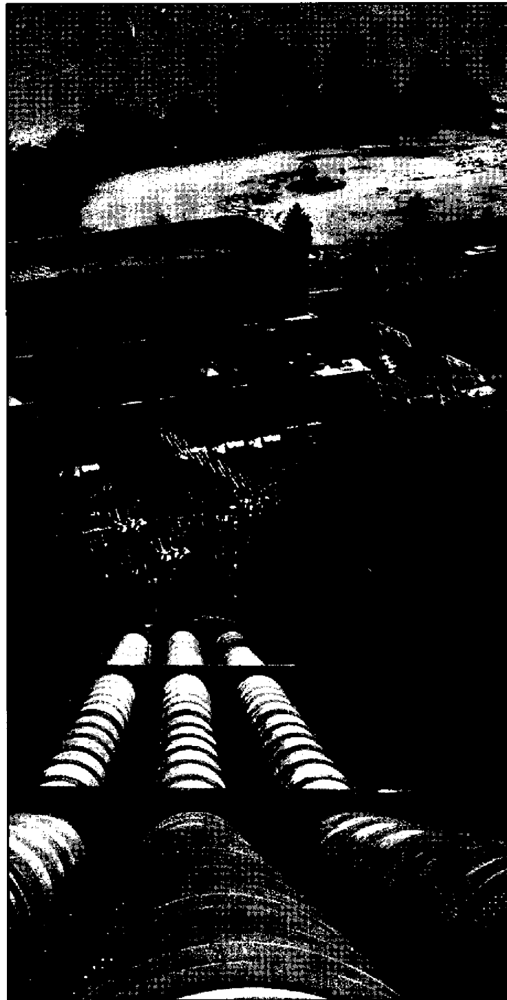
Large pipes carry rushing water from the impounded Skokomish River to the powerhouse below Cushman Dam.
